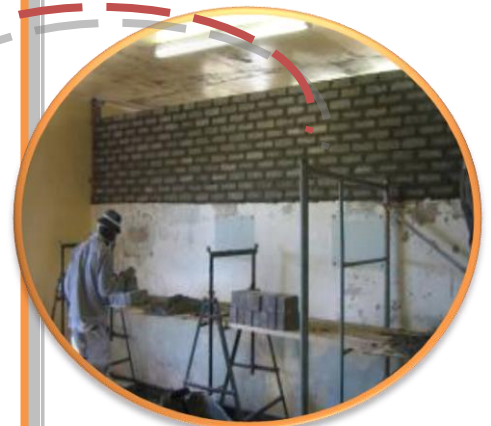
4. TB Ward renovation
